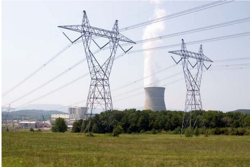
Nuclear power plant
