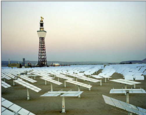
This 1996 photo shows the solar tower and surrounding field of mirrors for Solar Two, a demonstration project located near Bartow, California.
